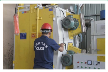
抛丸 Shot blasting
